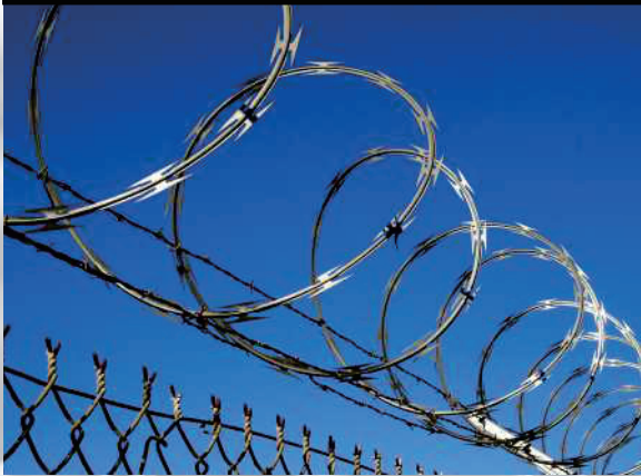
Concertina Wire & Chain Link Fence
