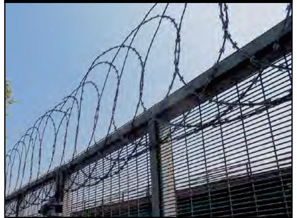
Topping of 358 Security Fence
