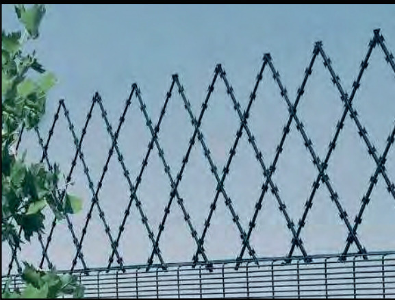
Razor Mesh on Fence Topping
