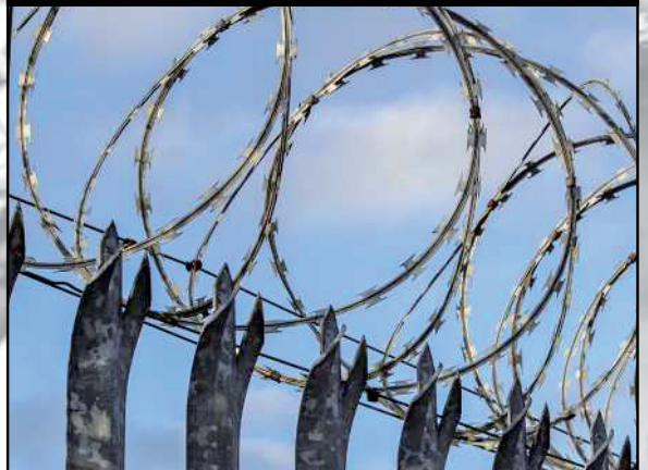
Concertina Wire & Palisade Fencing
